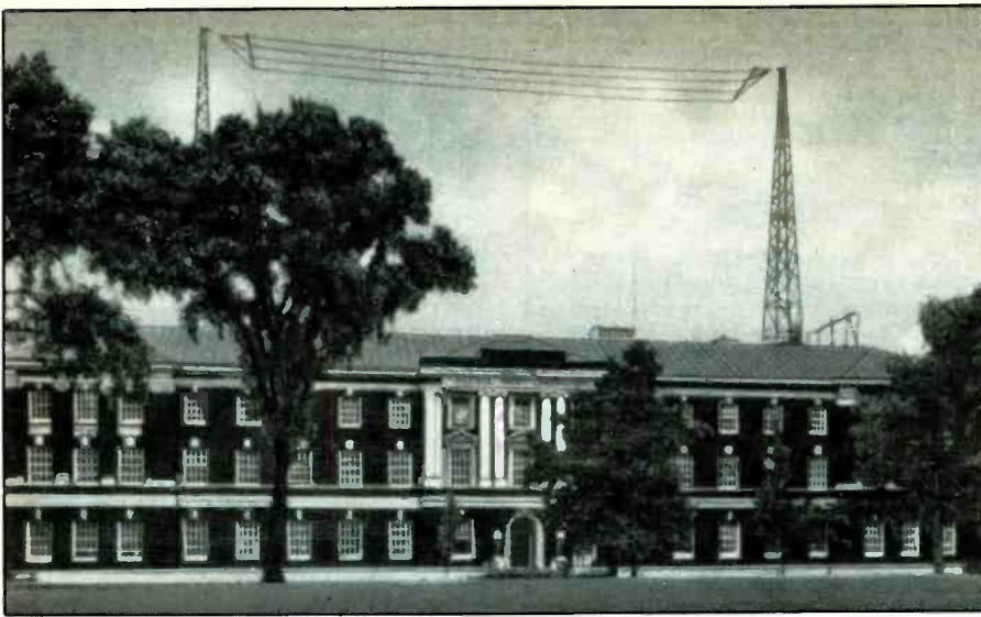
This view of the WHAZ antennas is probably from the 1940's. It shows the masts mounted atop the Engineering Building at RPI.
